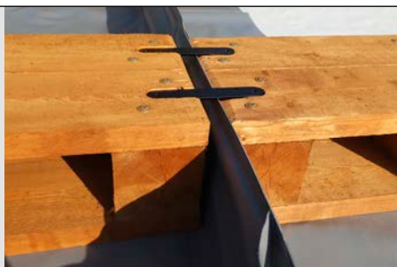
Detail of anchorage of a wooden ramp
